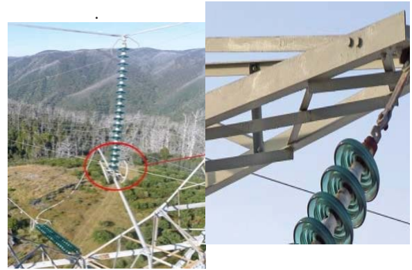
Figure 3- Two captured photo from cables and towers
