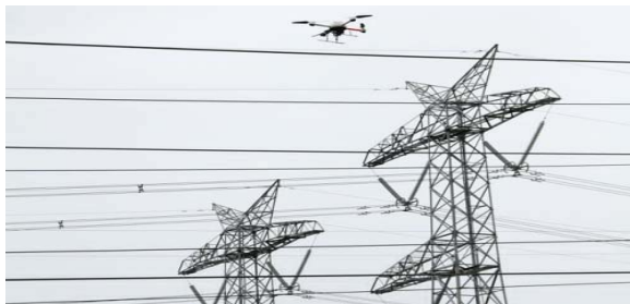
Figure 2- The UAV is inspecting pylons
